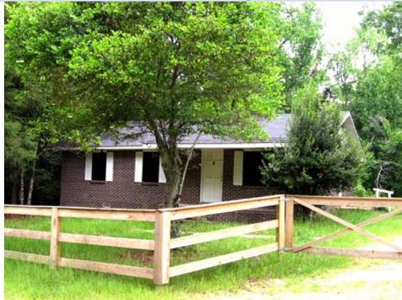
Front showing part of driveway gate
